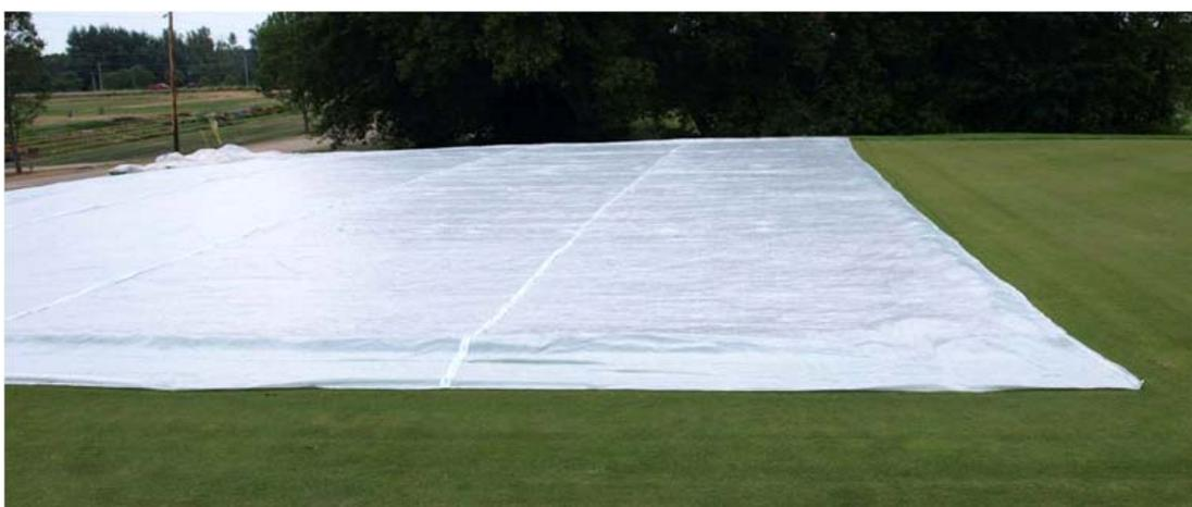
Figure 6. Permeable woven cover installed at seeding to stimulate germination and prevent erosion.
